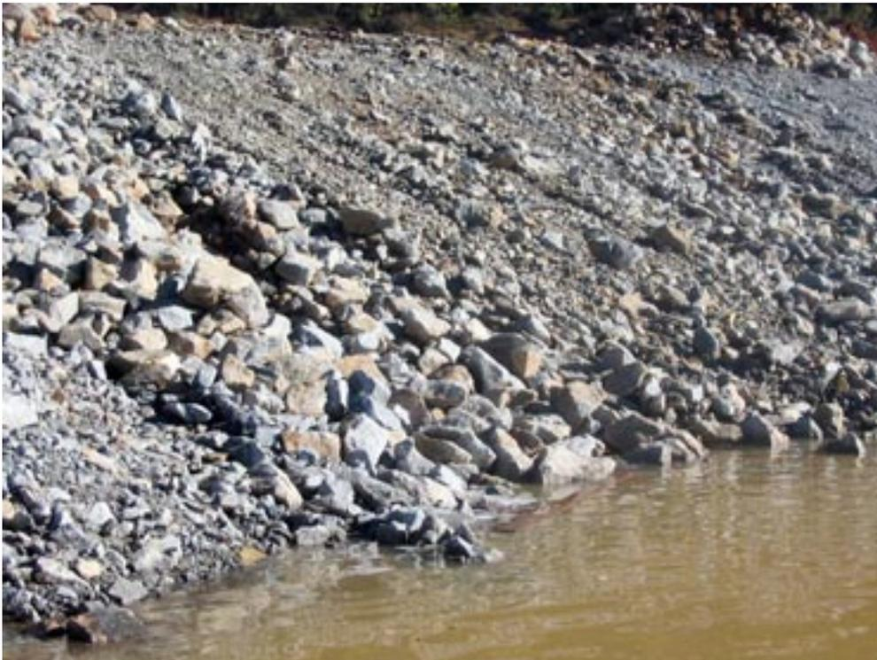
**Figure 23.** Inside view of the new wall of Lake Navarino showing the extension to the rock armour (to reduce the damage to the wall due to wave action). A). Extent of the new wall with the side extensions visible (as light coloured rock). B). Close up of the wall showing a large number of crevasses and holes.
